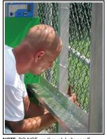
**NOTE:** DO NOT use through bolts or selftapping screws because you won't be able adjust the drive rail at a later date.
